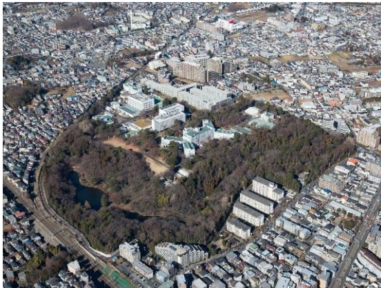
Aerial view of Kyōsō-no-Mori
